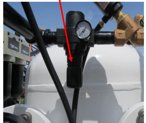
Pressure-regulator valve (screwing in, clockwise, increases the pressure)
